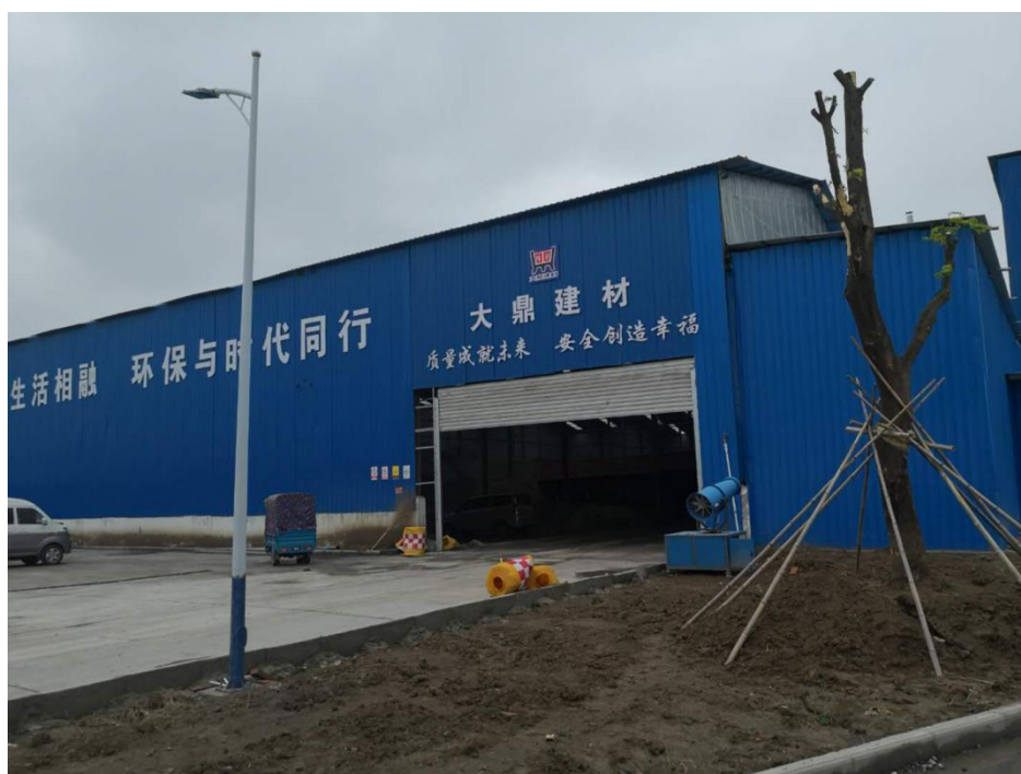
封闭式砂石料库
